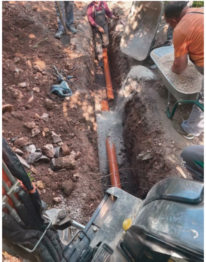
Photo 18: Improvement of the sewage installation, Neimari. d.o.o. Sarajevo
