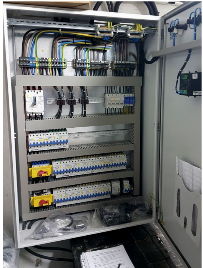
Photo 23: Replacement of the decrepit electric system, Ideologija, Sarajevo
