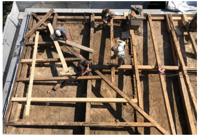
Photo 9 & 10: Restoration of the roofs above the Prehistory Section, Neimari. d.o.o. Sarajevo
