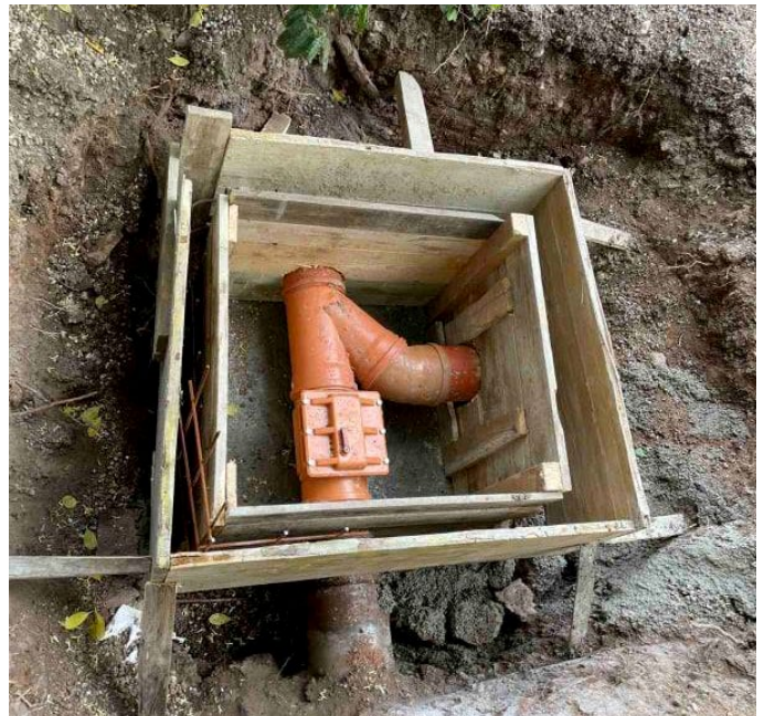
Photo 19: Improvement of the sewage installation, Neimari. d.o.o. Sarajevo
