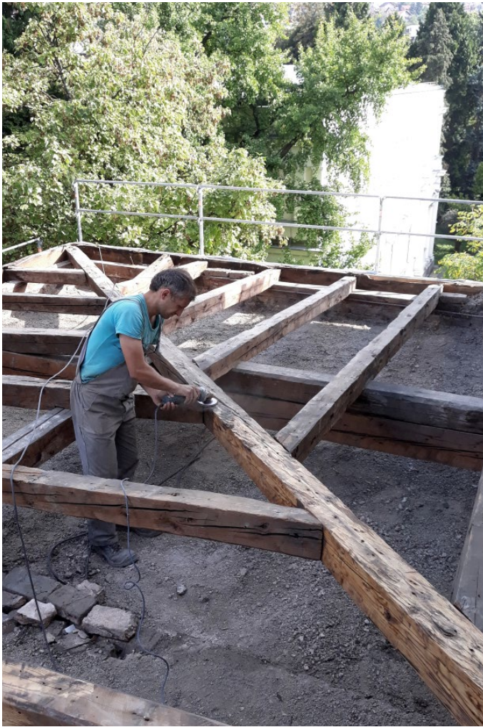
Photo 8: Restoration of the roofs above the Prehistory Section, Neimari. d.o.o. Sarajevo
