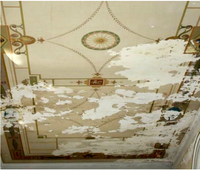
Photo 13: Restoration of the wall and ceiling paintings in the Prehistory Section, Commission to Preserve National Monuments
